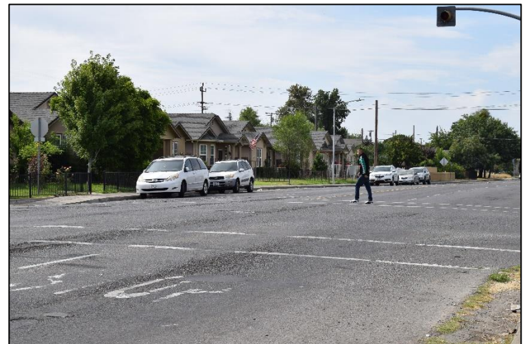
Faded condition of crosswalks along Rio Linda Boulevard.
