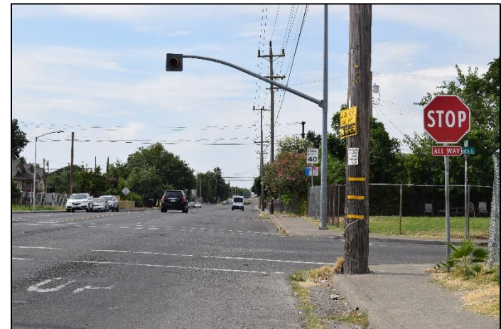
Example of intersection on Rio Linda Boulevard in need of crosswalk restriping, ADA compliant curb ramps, and other intersection improvements.
