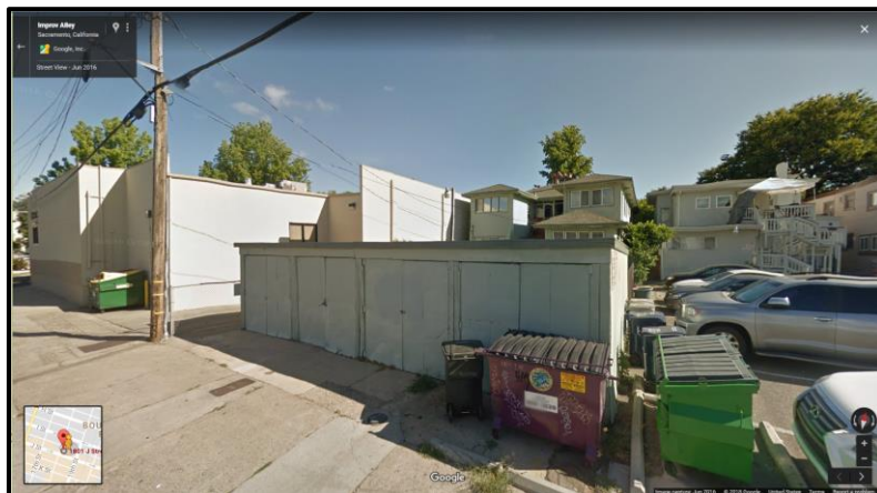
Figure 3 View of alley and adjoining properties to the north
