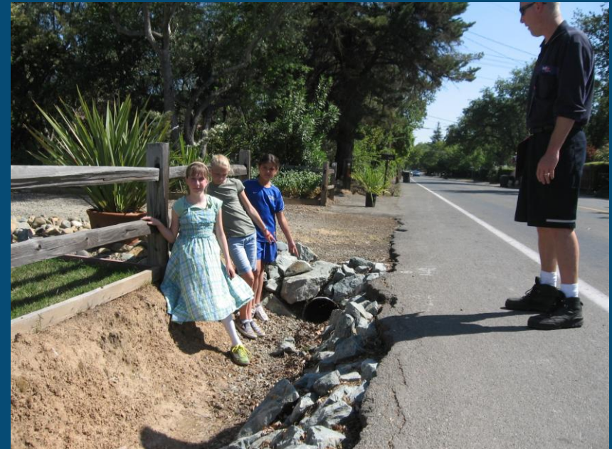
Ditch on California
