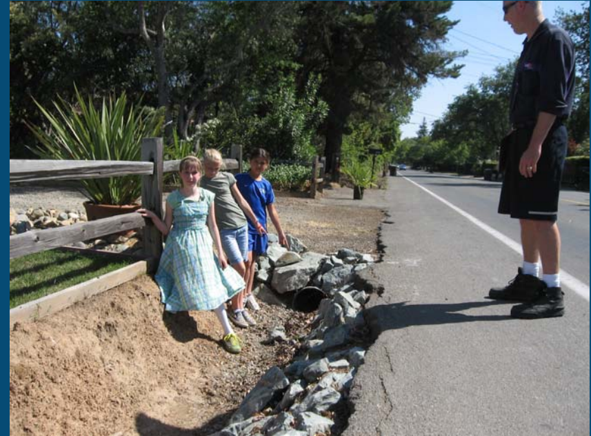
Ditch on California
