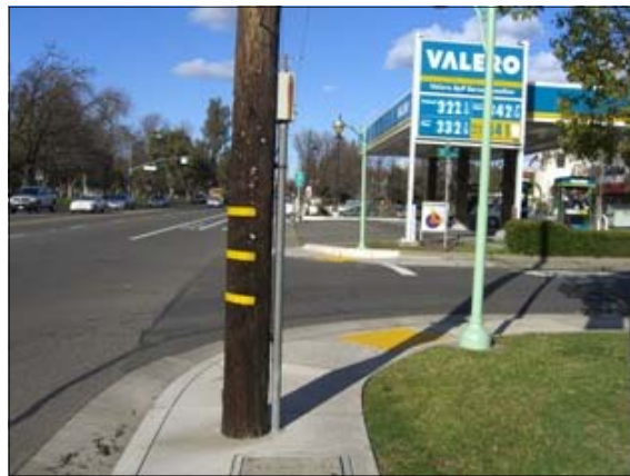
Curb cut with utility pole blocking sidewalk on Freeport Boulevard and 15th Avenue
