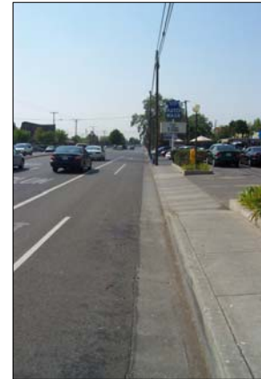
Freeport Boulevard looking south with unused on-street parking
