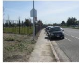
EXISTING CONDITION EAST SIDE
