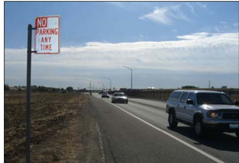
Lack of sidewalks around the campus perimeter, such as along Bruceville Road, pose a danger to pedestrians around and near the campus
