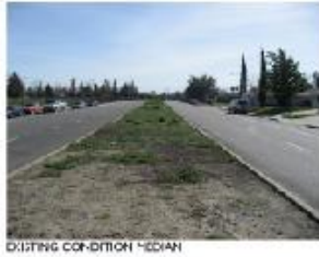
EXISTING CONDITION MEDIAN
