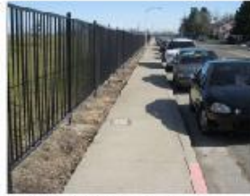
EXISTING CONDITION NORTH SIDE
