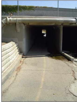
Florin Creek Trail undercrossing
