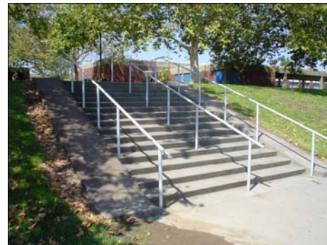
Steps leading to Cosumnes River College central campus level, an obstacle for bicyclists
